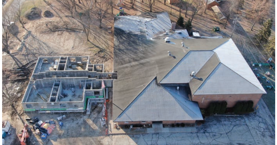
Thanks to CEF’s help, the foundation is set, and the walls are up for the new childcare wing at Immanuel.
